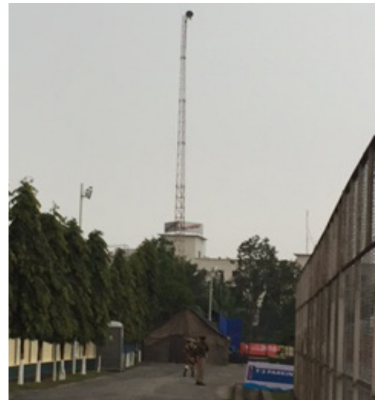
Tower for wireless backhaul link
